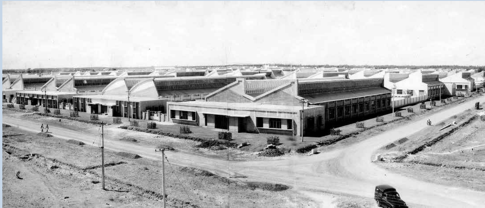
An early view of the Guindy Industrial Estate, courtesy The Hindu
