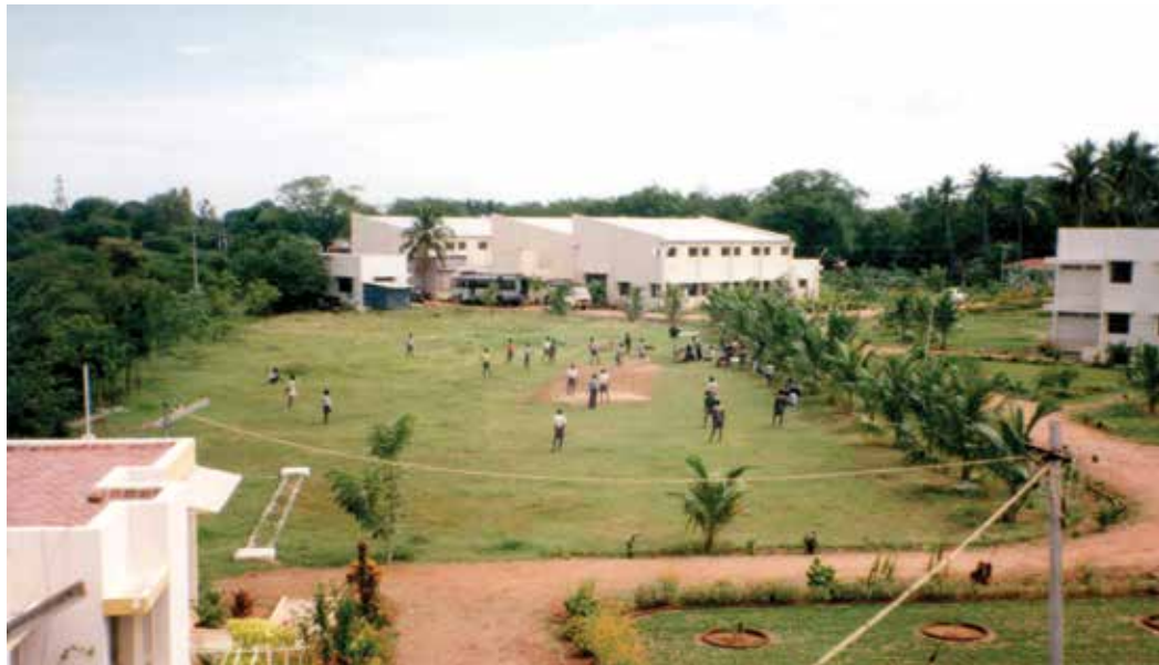
Production Centre at Trichy
